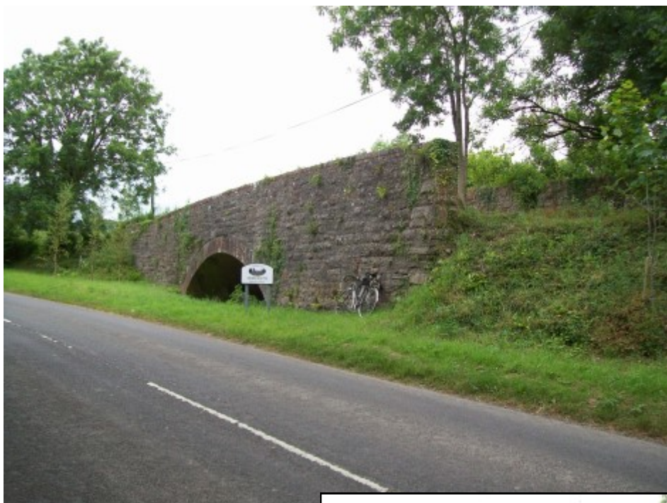
The bridge which carried the B3190 over the Barnstaple Branch near Morebath Junction is now partly filled in and bypassed.
