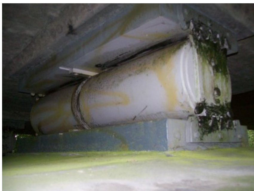
One of the two bearings at the top of each pier.
