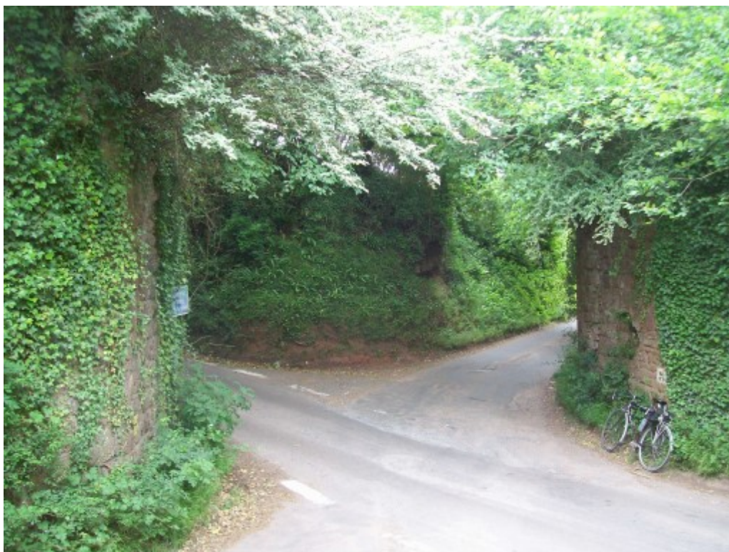
The ruined bridge at Croford was unusual in that it spanned a crossroads, perhaps a trick by the engineer to avoid realigning the roads or building two bridges.
